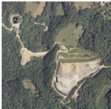
Fig. 1. Air picture of the Boršt tailings pile.
