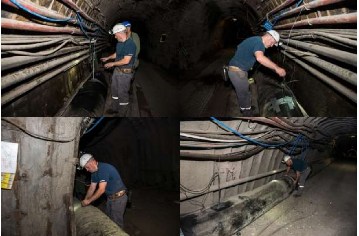
Figure 3.13: Final inspection and setup of ducting and sensors.
