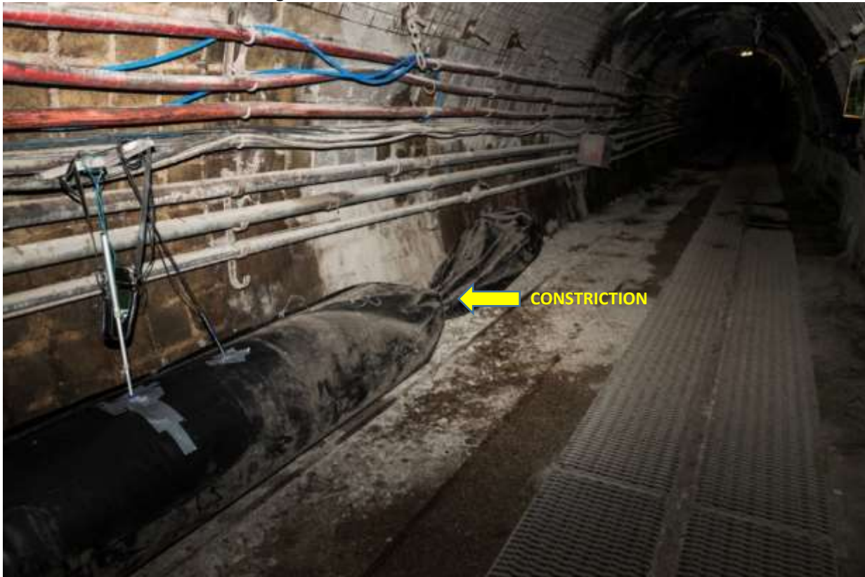
Figure 3.14: View of the end of the ducting layout with part of the layout of monitoring location 2 in the airway with the cross-section reduction or constriction, respectively.
